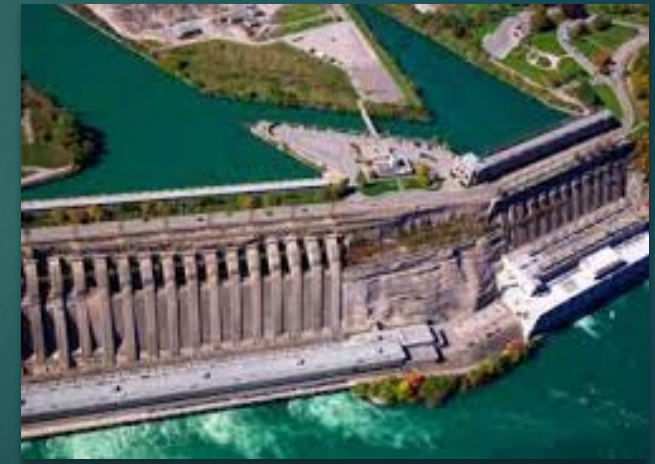
Robert Moses Niagara Power Plant and the Lewiston Pump Generating Plant in Niagara Falls generates 2.6 million kw of clean energy annually.
